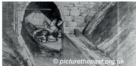
“Legging” through Cromford canal tunnel 1845
