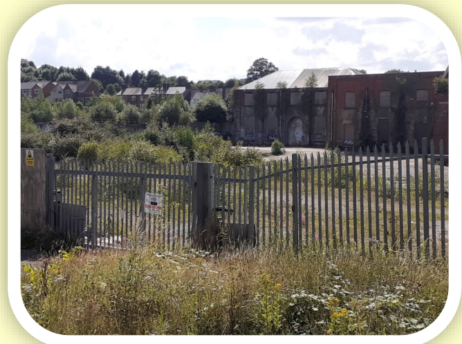
Former Butterley Ironworks site in Ripley
