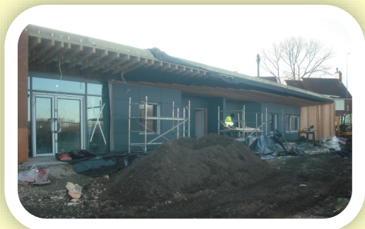
The new community facility at Greenwich Park
